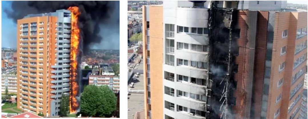
Figure 8 – The Mermoz Tower in Roubaix, France, during and after the 2012 fire (Youde, 2017)
