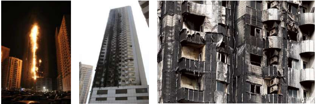
Figure 6 - The Al Tayer Building in Sharjah, Dubai, during and after the 2012 fire (Emirates 24/7, 2012; 2012b; Baldwin & Leon, 2012)
