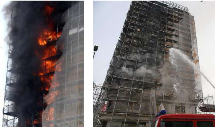
Figure 11. Toxic gases released from the burning façade made of EPS
